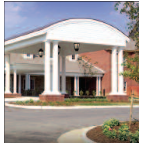
Exterior of main building at The Glebe
